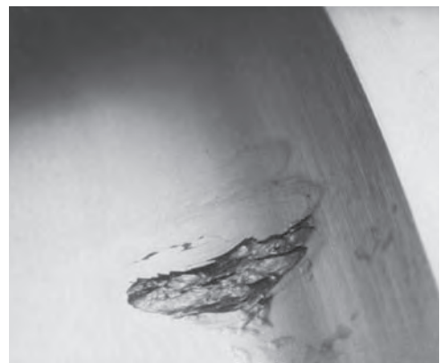
Fig. 5.2 Photo-illustration of fatigue damage on the raceway
